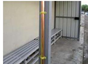
Pipe clamp for gas black coated M6 with chipboard screw
